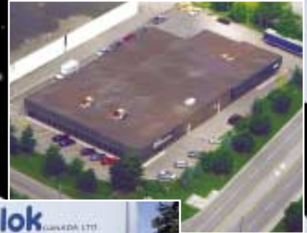
NIMLOK CANADA, CANADIAN HEADQUARTERS
